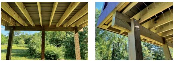
Notched 6x6 posts with double or triple 2x10 beams using a thru-lock system to tie the beam and posts together.
